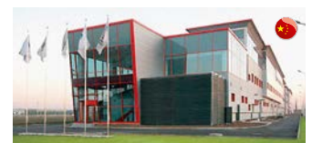
ARNOLD FASTENERS SHENYANG Shenyang China
